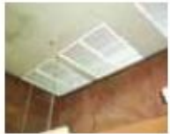
Push Hood Sends filtered clean air into the room.
